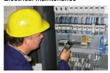
Infrared thermometers are proven time saving tools for predictive maintenance of electrical systems. Check out temperature problems safely with connectors, fuses, electric motors, motor windings, insulations, electrical wiring and electrical cabinets before damages occur.
