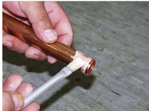
4. Apply the soldering flux on the pipe
