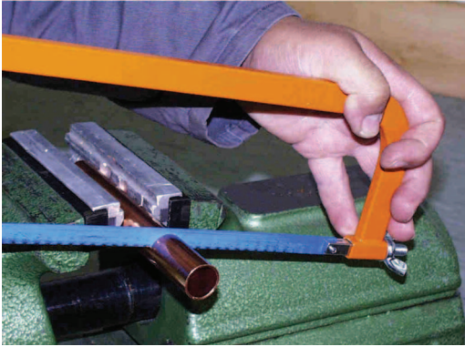
1. Rectangularly saw off the pipes
