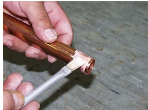
4. Apply the soldering flux on the pipe
