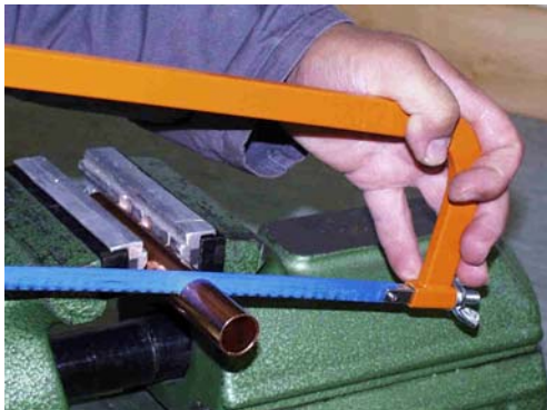
1. Rectangularly saw off the pipes
