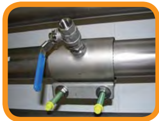
Spot drilling collar
